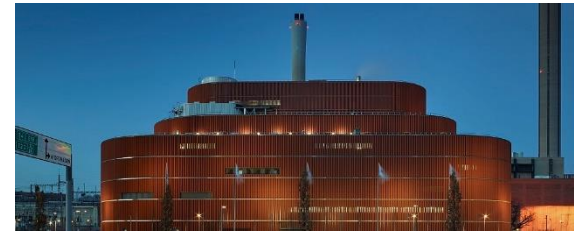
Combined Heat and Power (CHP)
